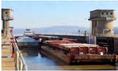
Hydroelectric Facilities: Large Rotating Equipment
