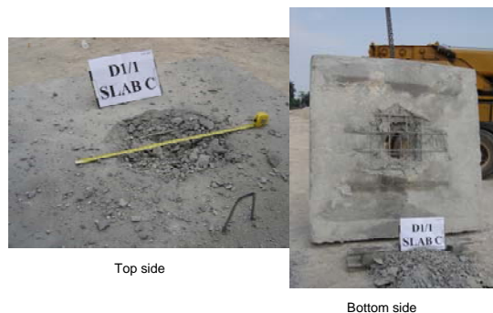
Fig. 4: Damage pattern for 2Kg TNT from test
