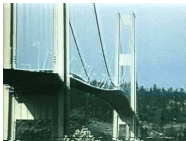
Tacoma Narrows Bridge, USA (Collapse 7.11.1940)
