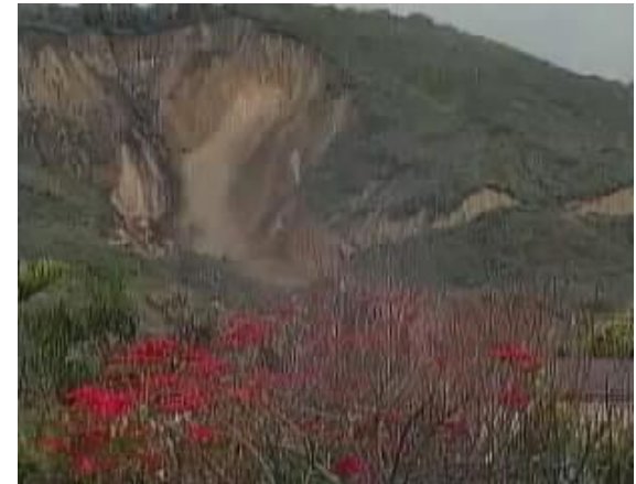
[The 2005 La Conchita Landslide]
